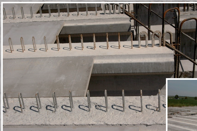
BETONYP® as formwork
