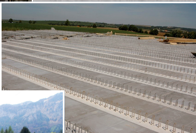
BETONYP® as formwork
