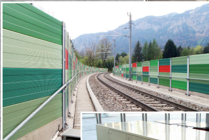
BETONYP® as noise reduction wall
